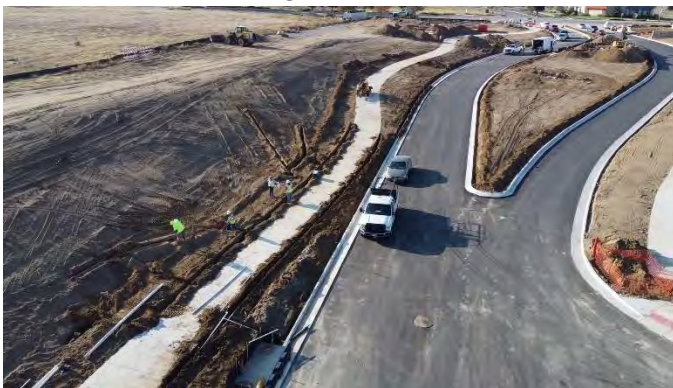
S. 35 th Ave Utility Installation
