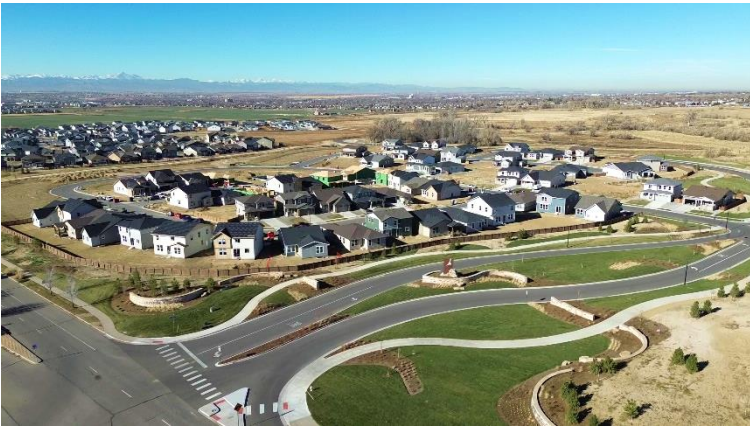
Overall View – Facing Northwest
