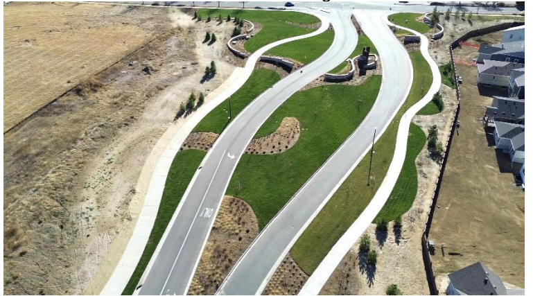
Entrance Landscape Improvements – Facing South
