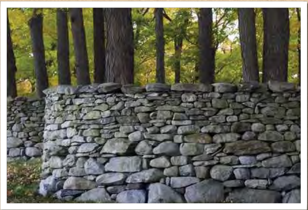
Artful gradation application from large sized stone to smaller sized stone from bottom to top.
