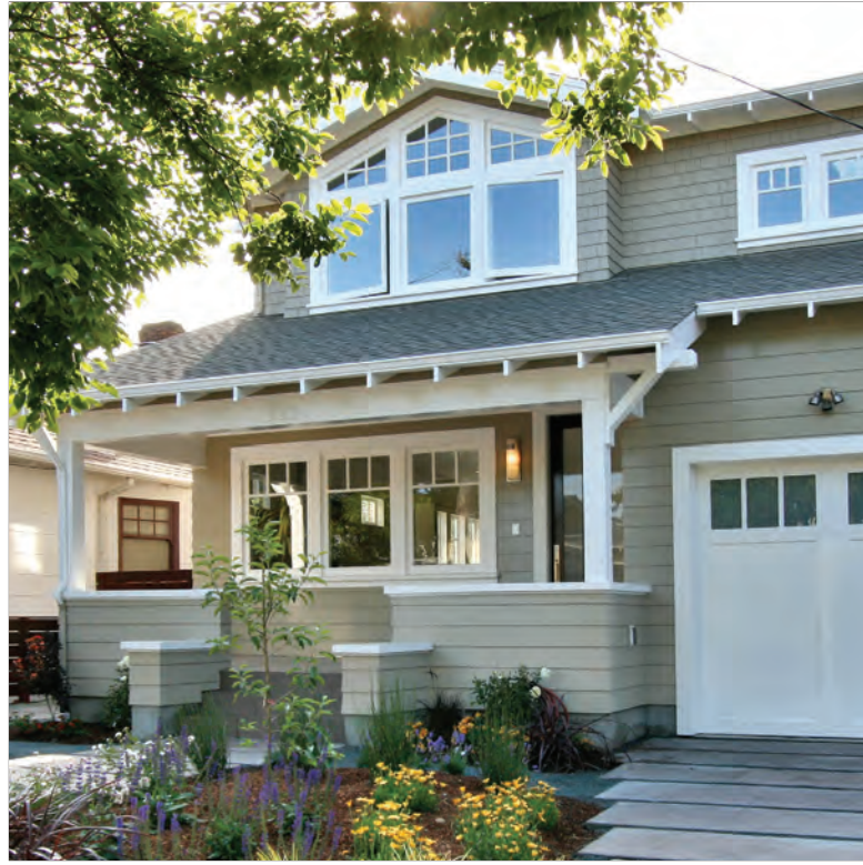
Low pitched craftsman-style gabled roof forms with large overhang and exposed rafter tails.
