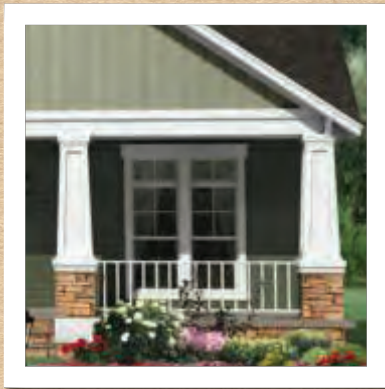
Stone base with battered craftsman column with reveal
