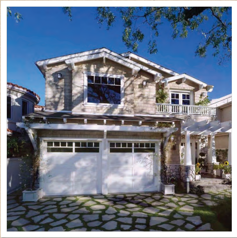
Low pitched craftsman-style gabled roof forms with large overhang and exposed rafter tails.
