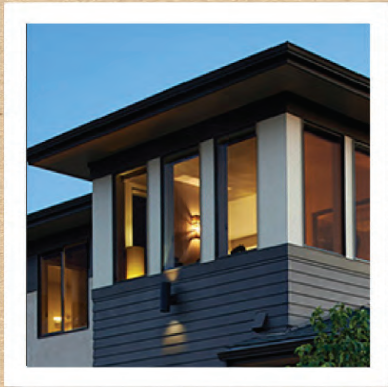
Low pitched prairie-style hipped roof form with large soffited overhang.
