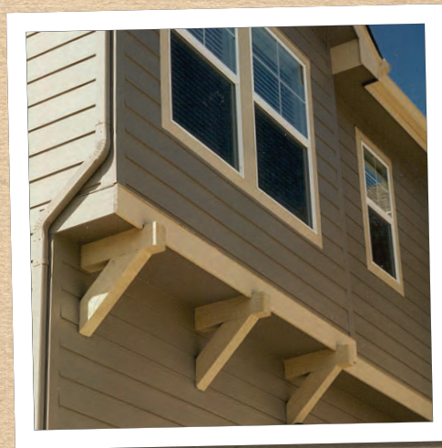
Craftsman support brackets create an anchored building projection.
