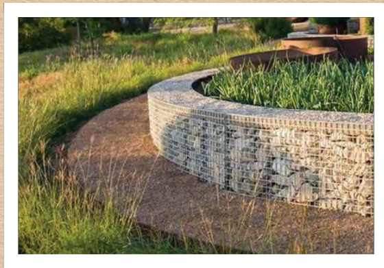
Freestanding gabion wall with rough filled stone
