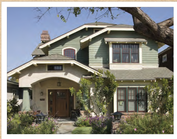
Craftsman style roof with exposed rafter tails and generous overhangs.
