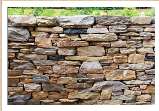
Dry stacked stone retaining wall
