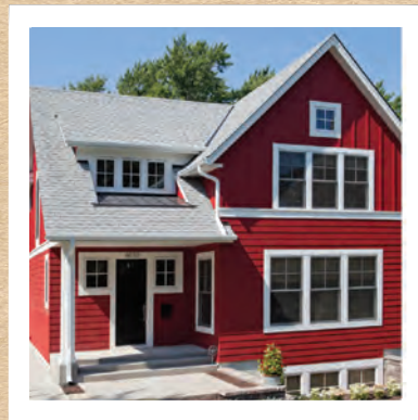
Simple front-falling gable roof and shed dormer
