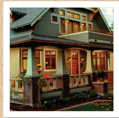
Thick and wide craftsman column with masonry base
