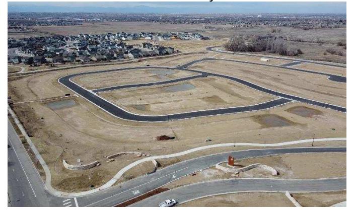
Overall View Facing West
