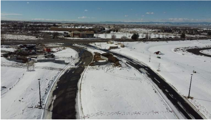
S. 35 th Ave Median Work In Progress
