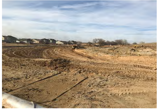
Over Excavation Southwest
