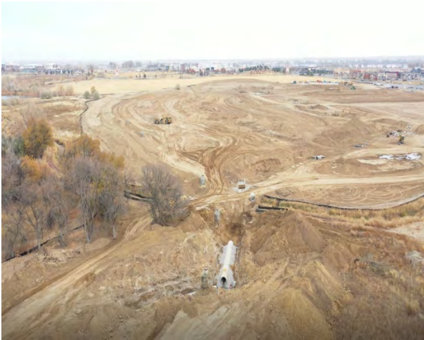
Storm sewer creek crossing and grading
