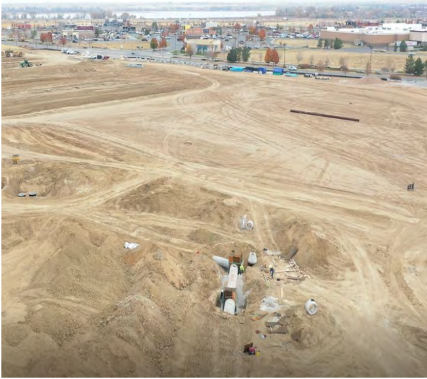
Storm sewer and grading
