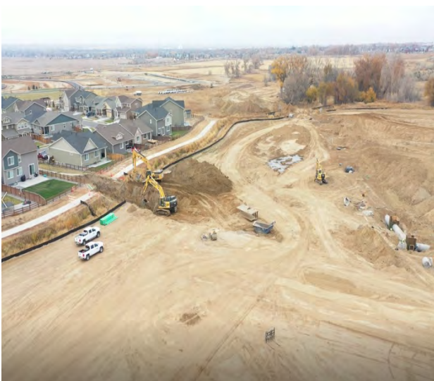
Grading and sanitary tie in
