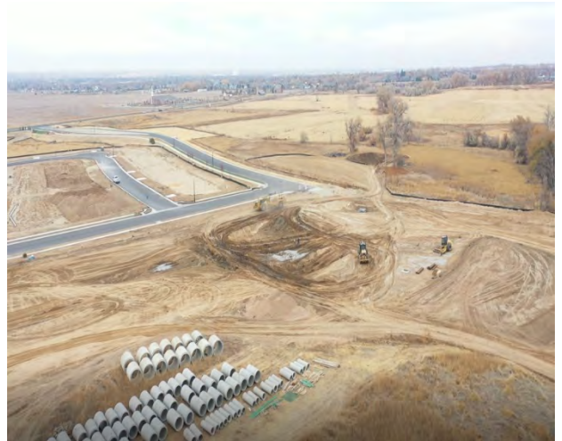
Grading and material storage
