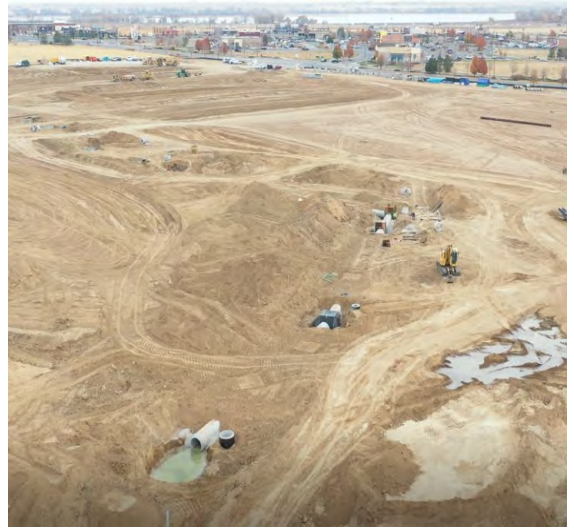
Storm sewer and grading
