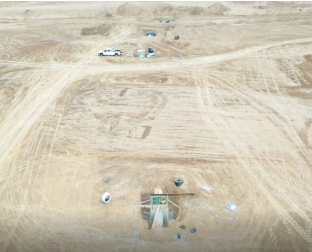
Storm sewer and grading
