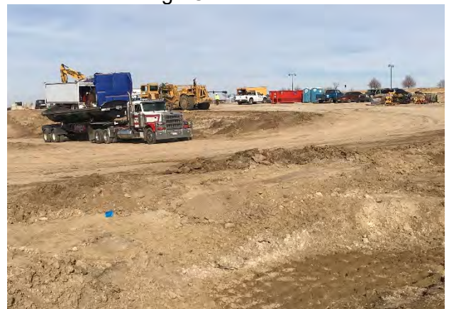
Site Entrance and Staging
