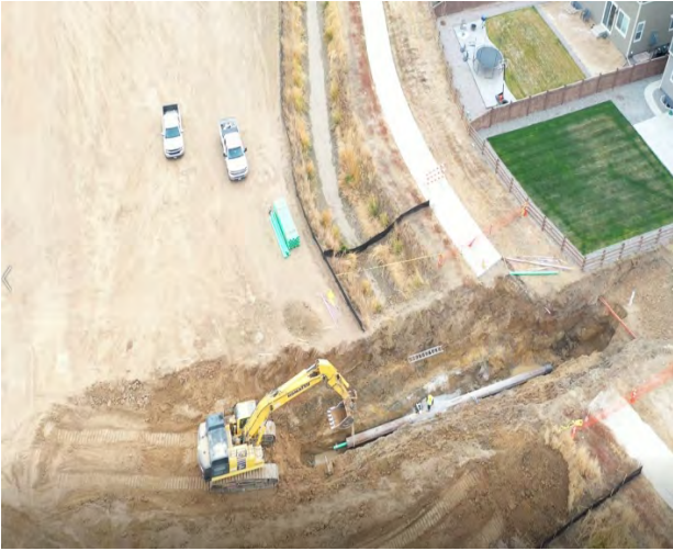
Sanitary main tie in
