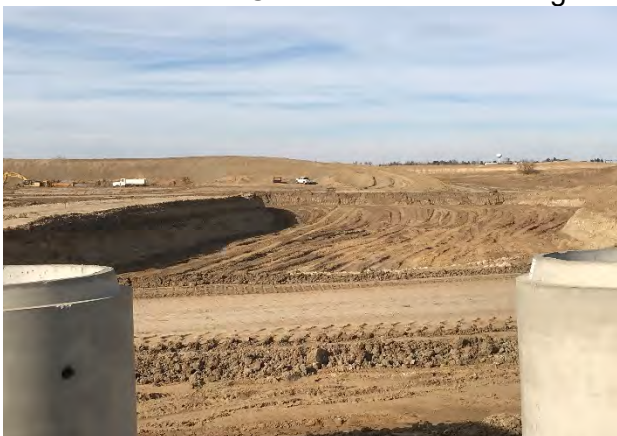
Over Excavation South
