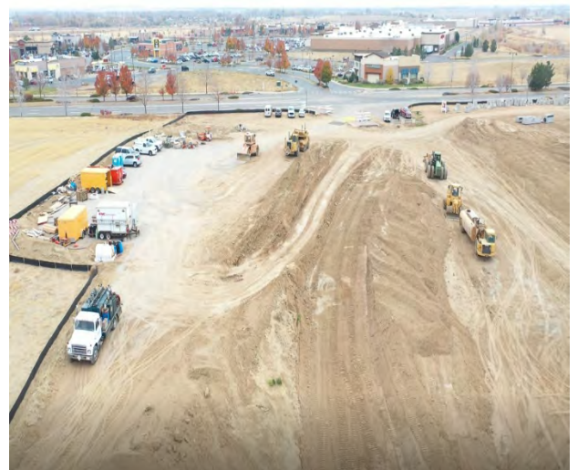
Staging and site entrance
