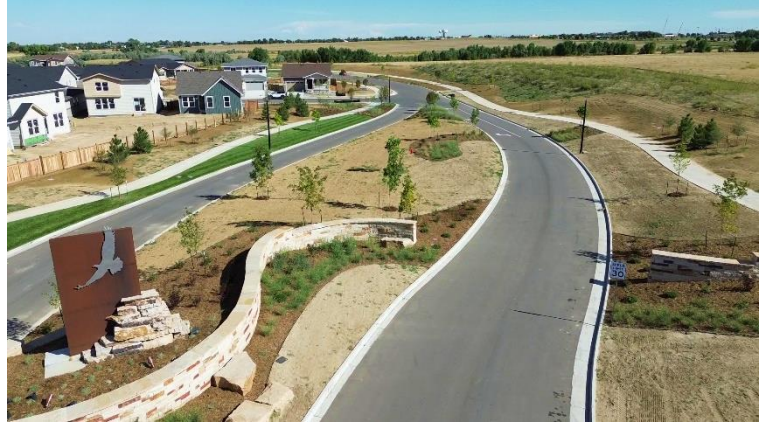
Landscape Improvements along Median – Facing North
